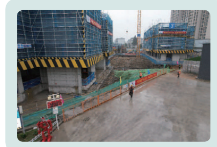
場地硬化、定型欄桿 Site hardening, and standardized guardrails
