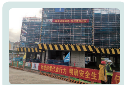
施工圍護、安全標語 Construction fences and workplace safety slogan
